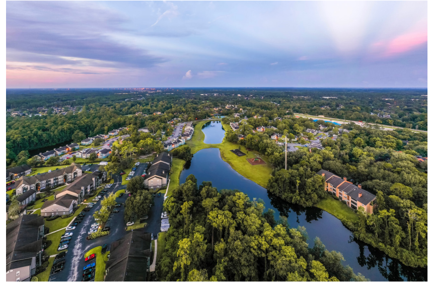
The Antlers Apartment Homes aerial view
