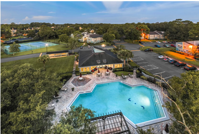
The Antlers Apartment Homes pool and clubhouse
